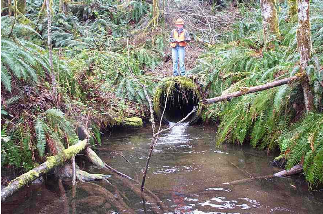
Figure 29. Outlet of railroad culvert MP 12.73.
