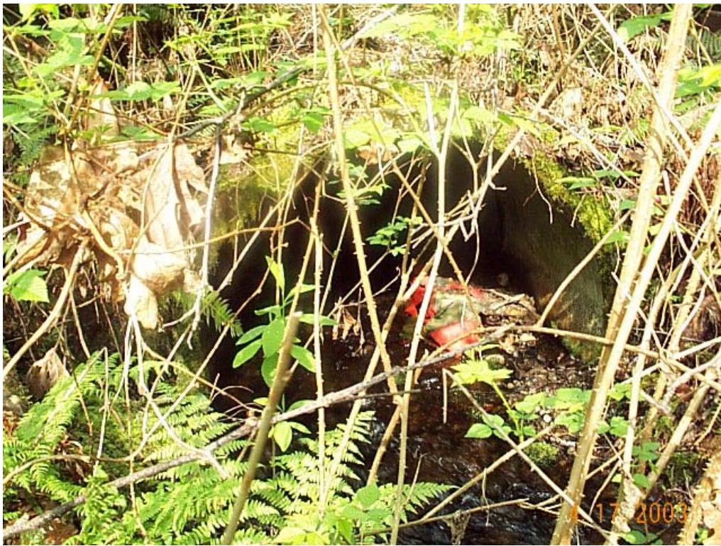
19. Outlet of railroad culvert MP 7.52.
