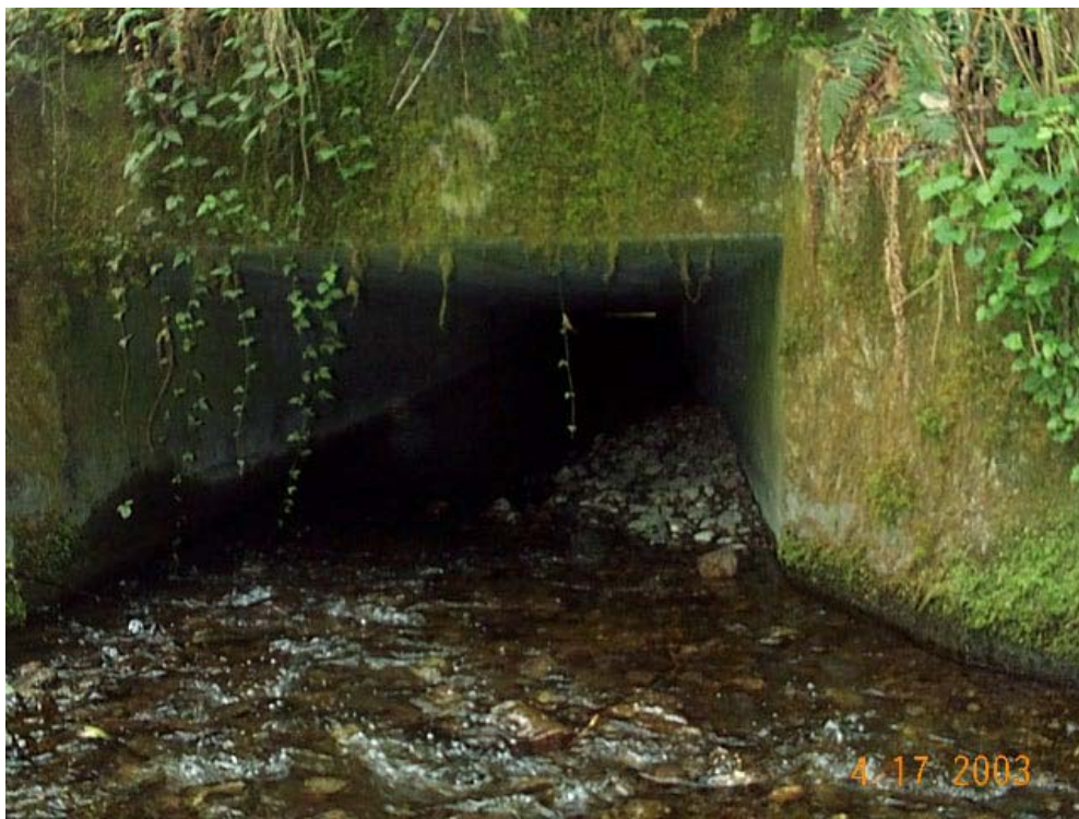
Figure 40. Inlet of railroad culvert MP 31.55.
