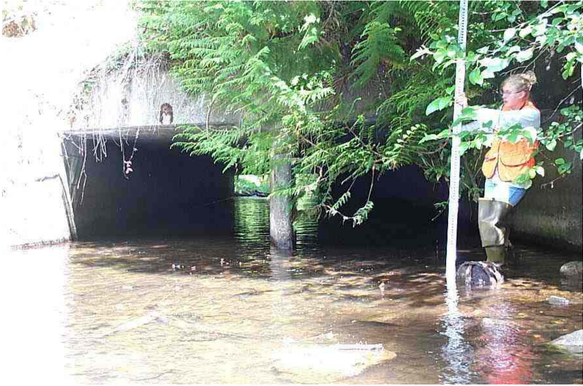
Figure 18. Cranberry Creek box culvert, railroad MP 6.60.
