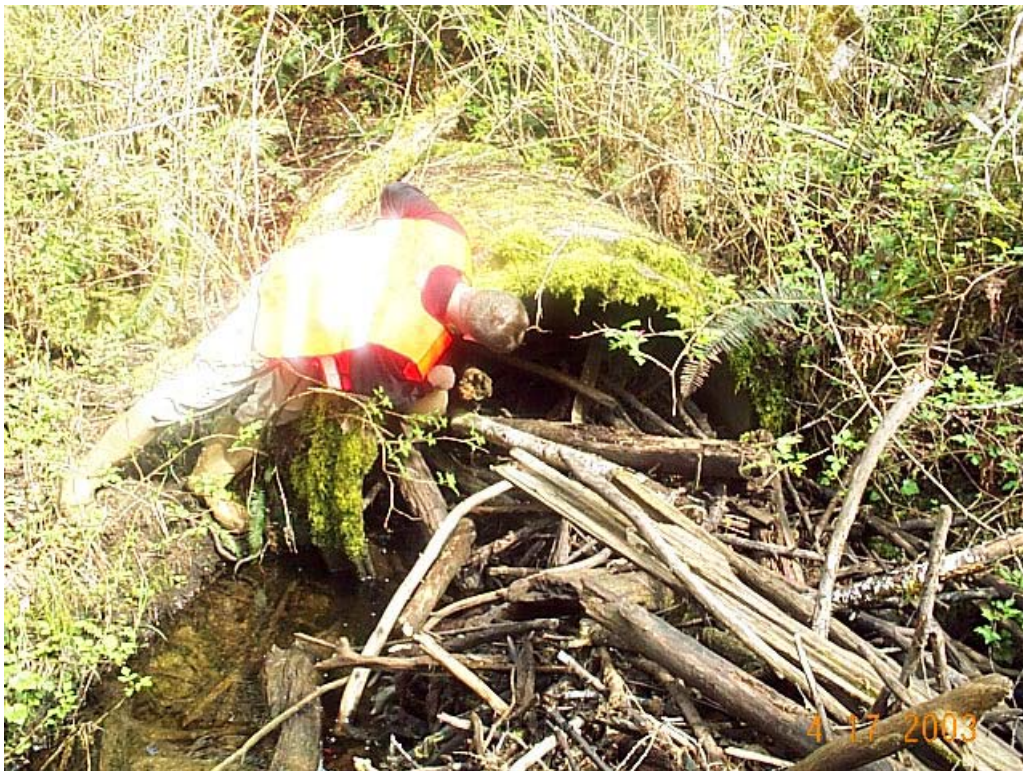
Figure 27. Outlet of railroad culvert MP 12.01.
