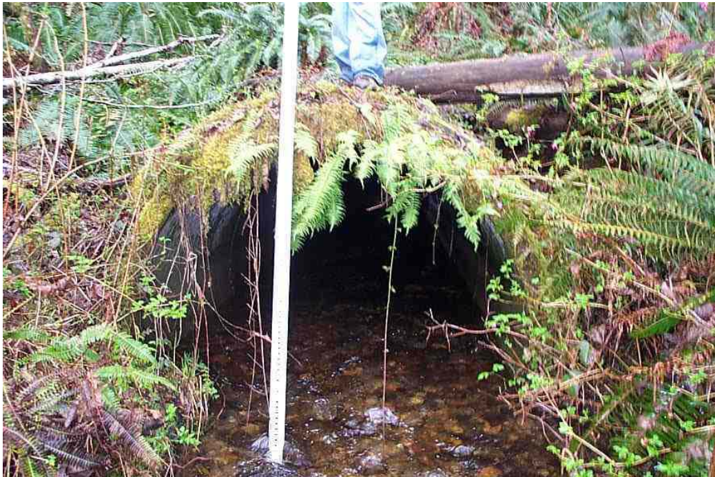
Figure 22. Outlet of railroad culvert MP 9.28
