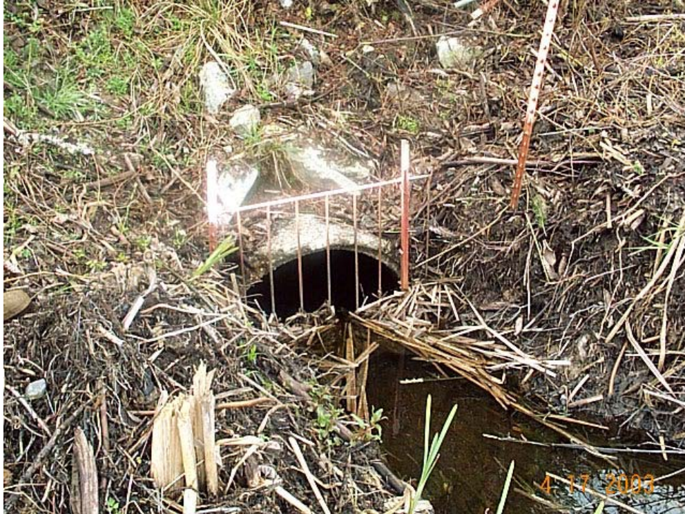
Figure 24. Inlet of railroad culvert MP 10.50.
