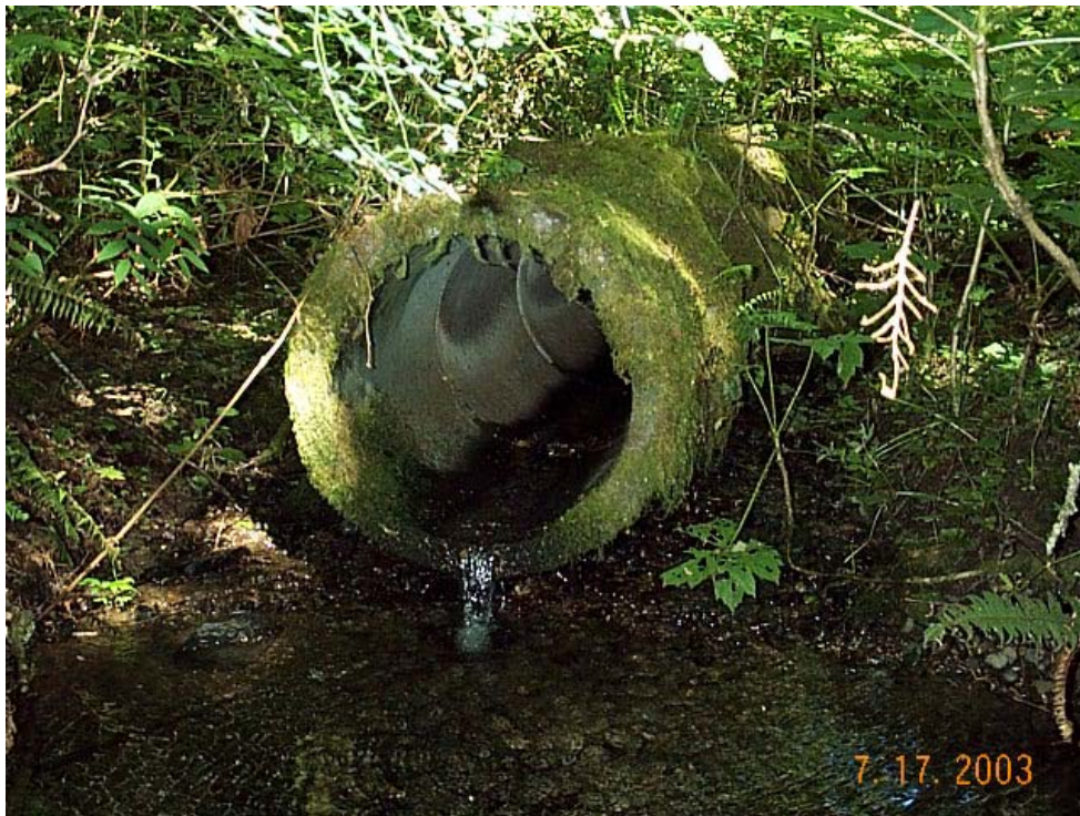
Figure 48. Outlet of Jarstad Creek (railroad MP 1.04) culvert.
