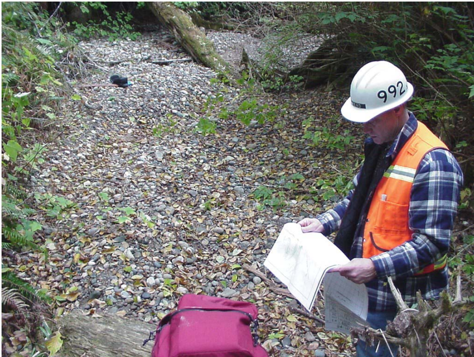
Figure 37. Inlet of railroad culvert MP 28.24.
