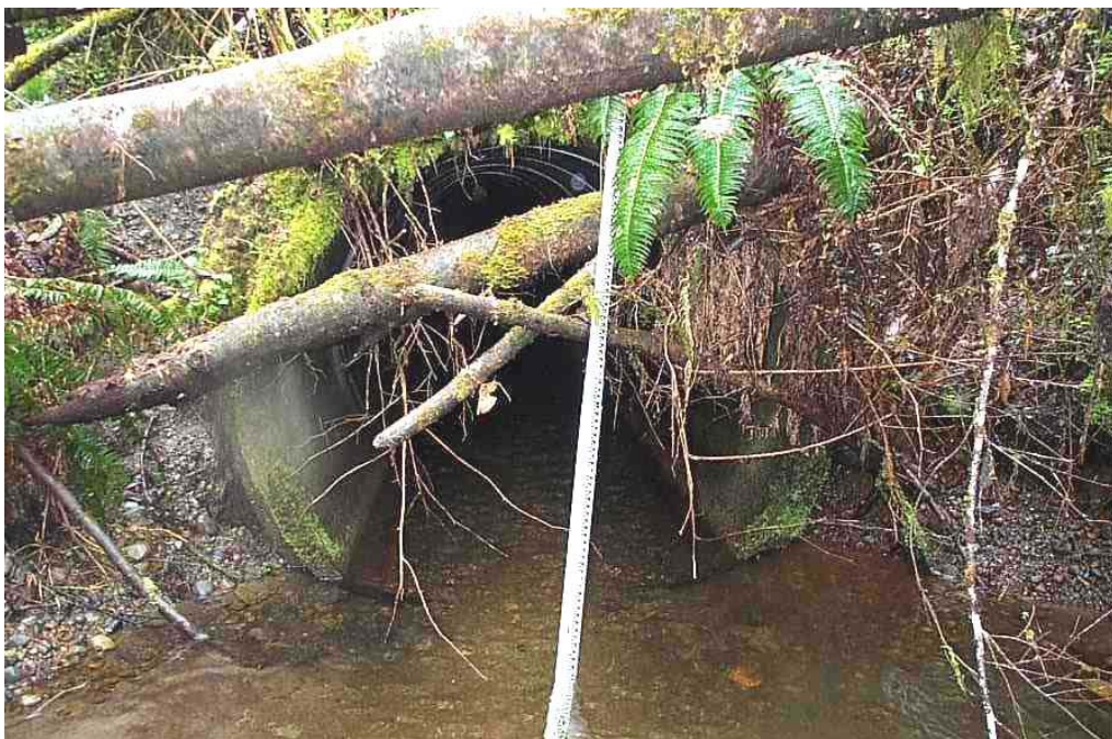
Figure 21. Outlet of railroad culvert MP 8.90.
