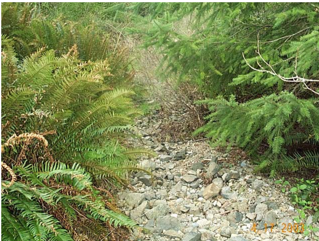
Figure 43. Outlet of railroad culvert MP 32.09.
