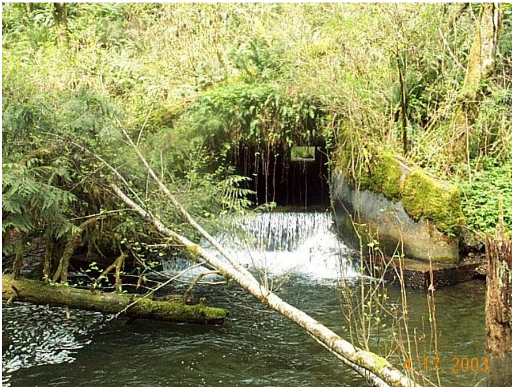
Figure 45. Heins Creek (railroad MP 0.71) culvert outlet.
