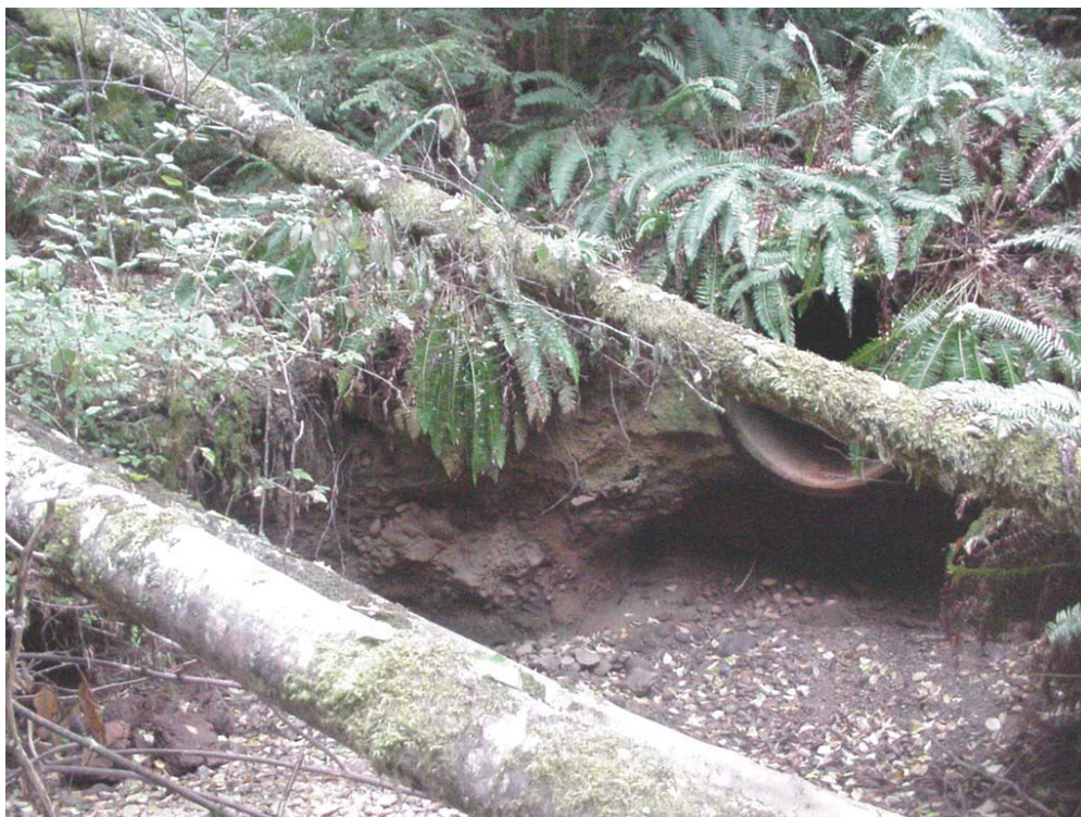
Figure 39. Outlet of railroad culvert MP 28.24.
