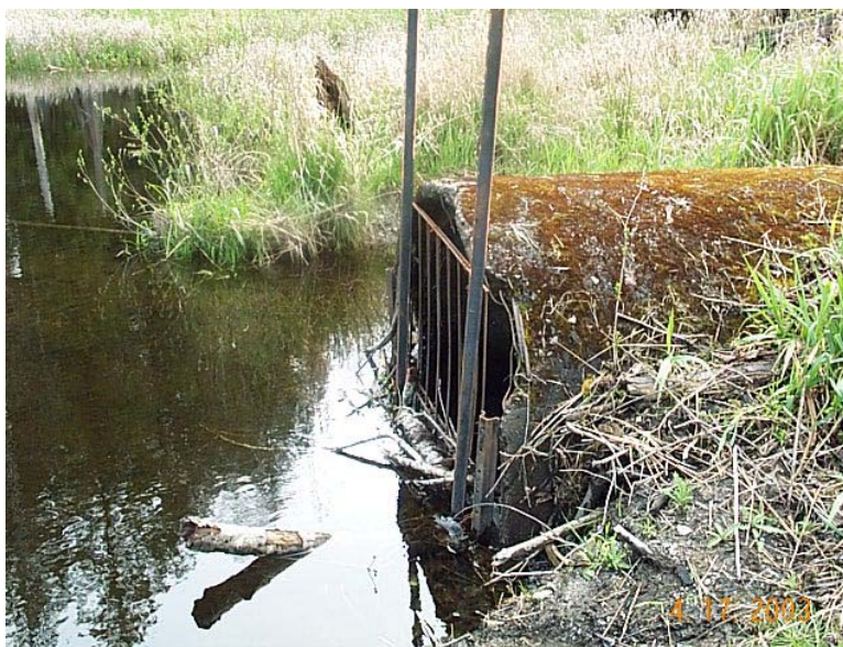
Figure 25. Existing inlet of railroad culvert MP 12.01.
