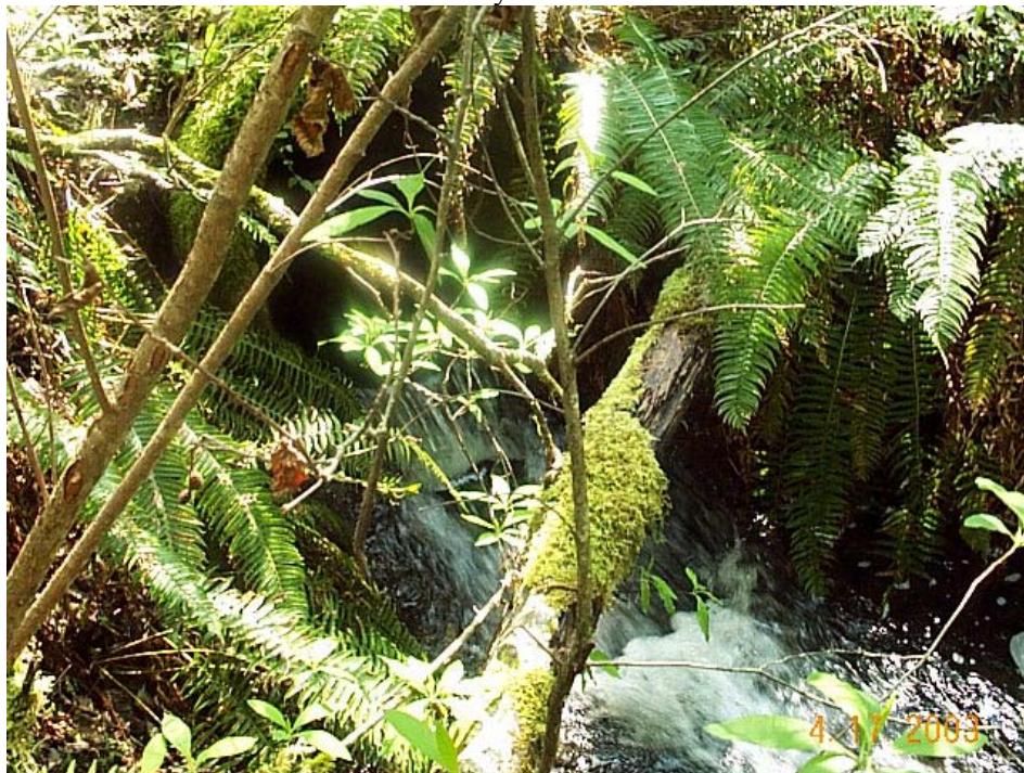
Figure 35. Outlet of railroad culvert MP 21.67.
