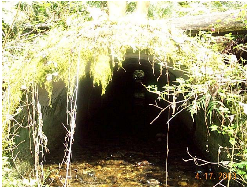
Figure 32. Outlet of railroad culvert MP 13.10.
